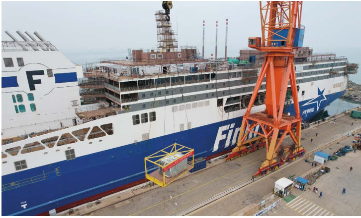
The cabin installations of Finnsirius took place in autumn 2022.
